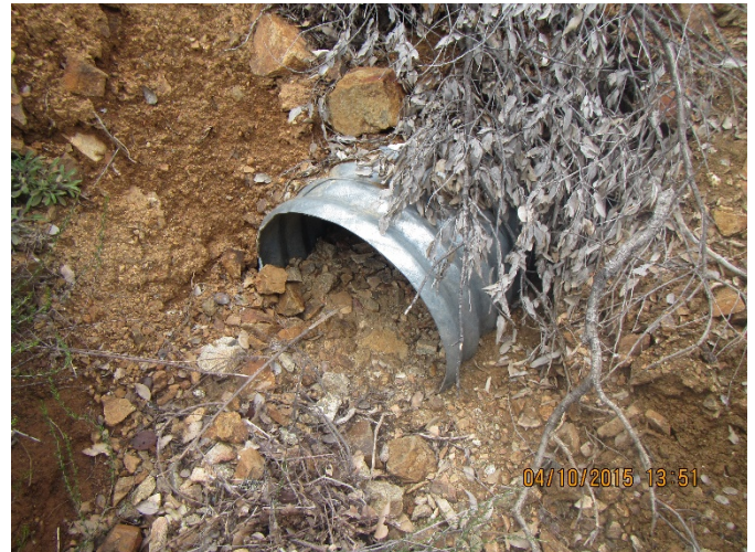
Photo 10 (Mustain) – C4 Partially Plugged Outlet
