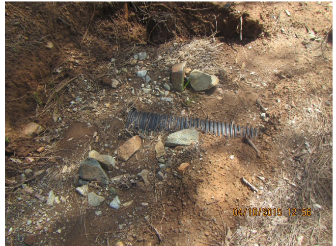
Photo 4 (Mustain) - Buried Ditch Relief Culvert
