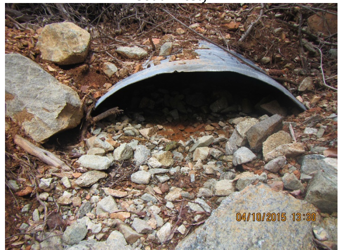
Photo 8 (Mustain) - C3 Plugged/buried Outlet (Facing Northeast)
